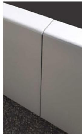
The top edge of each element ends in a fold and a counter-fold. The connection between each module is made on a straight edge of sheet metal, without a fold, by means of a joint plate. The fasteners are not visible on the external faces and are secured by means that avoid the risk of galvanic corrosion. Vertical ribs reinforce each element at the end and additional reinforcements are added to maintain the rigidity of long modules.
